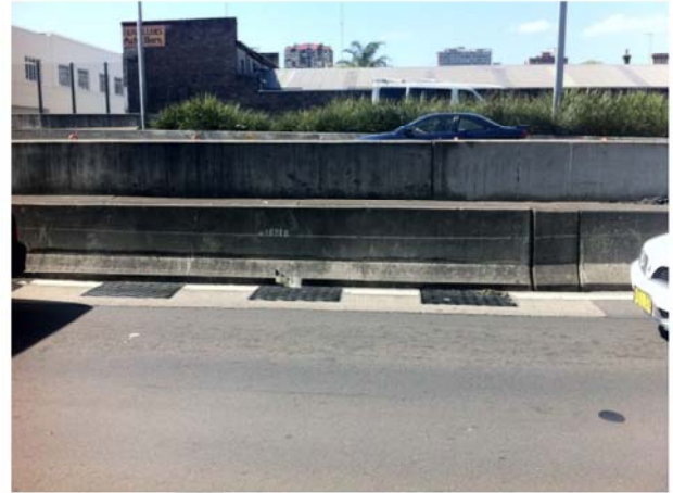
Photo 18: 4x0.6x1.0 m grated inlets
