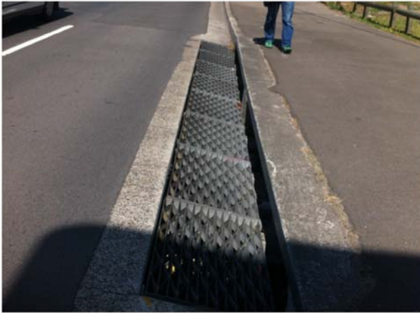
Photo 17: 7.2m lintel and 7x0.6x1.0 m grated inlets
