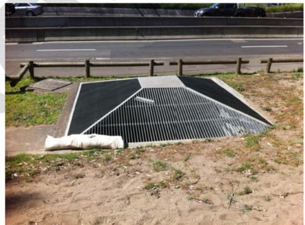
Photo 16: 4 m by 4 m inlet pit
